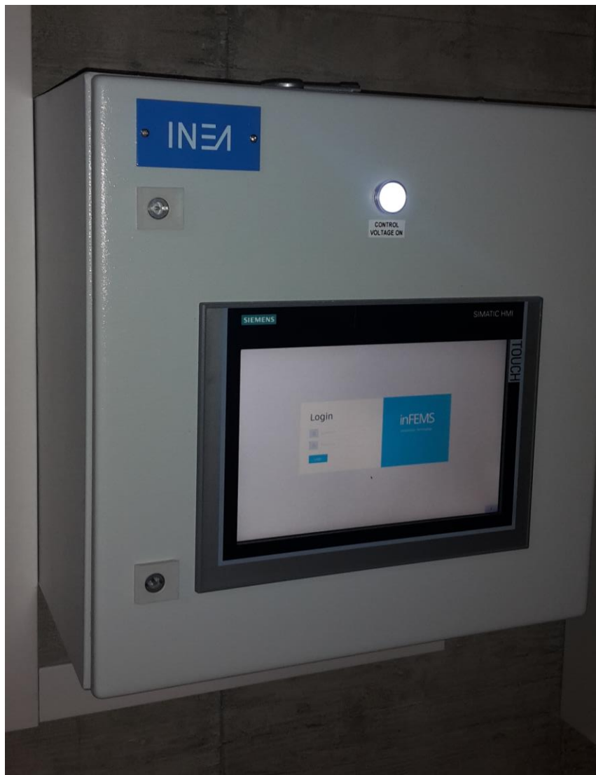
Figure 25 - FEMS cabinet installed at FEMS 8
