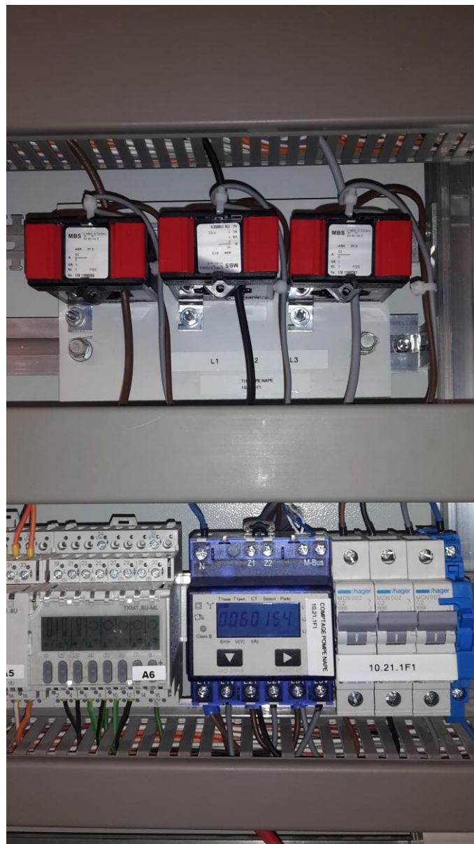
Figure 26 - A power meter installed at FEMS 8 with the split-core current transformers
