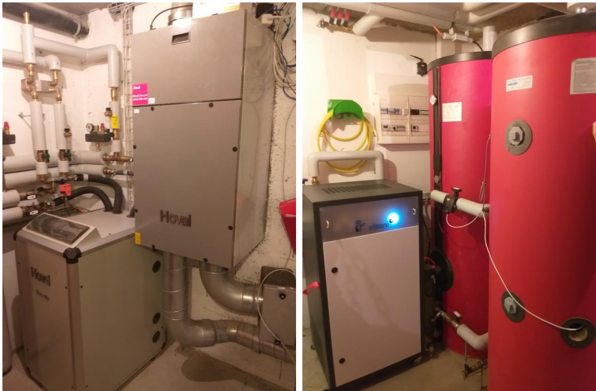
Figure 34 - The first installed CDEMS including a heat pump (left), two water tanks for space and water heating (right) and the deployed battery (right)
