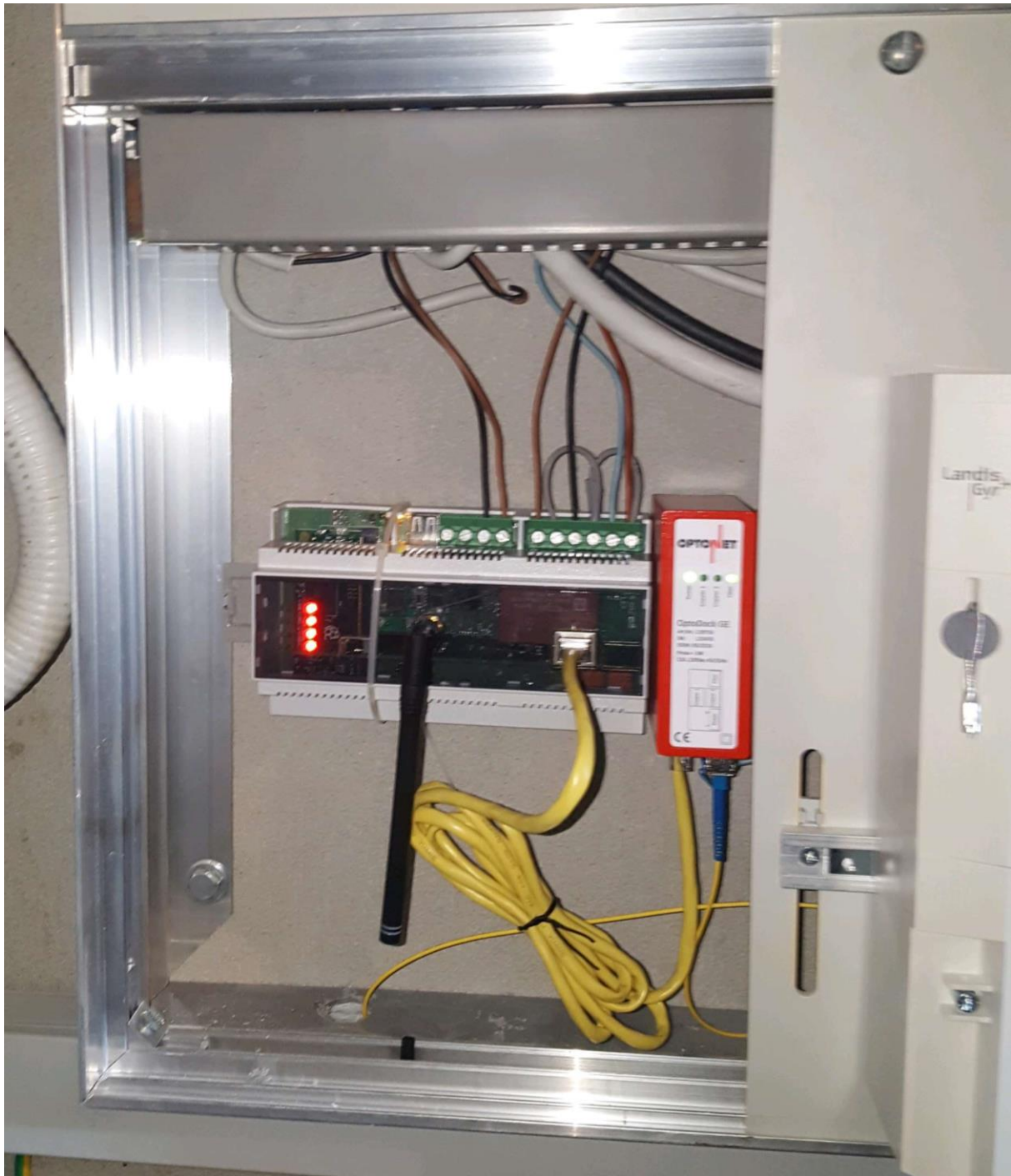
Figure 44 - Near final version of the Gateway connected to the optical fibre modem.
